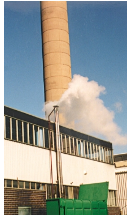
Steam plume before project (See also page 6)
